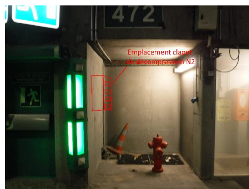
Figure 23 - Localisation clapets de ventilation
